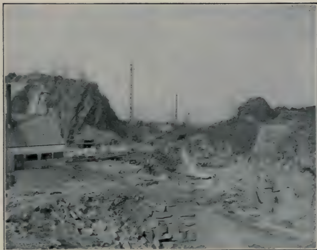
TOP OF INCLINE, GRANITE RAILWAY QUARRY, QUINCY, MASS.
